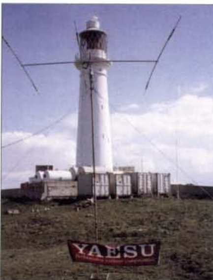
Fig. 1: The 3-element Tri-band antenna at 30ft (9m) sitting on top of a copper ground mat installed years ago by Trinity House as there was a radio beacon at this point once (which is now gone but the mat remains). The beam is only 100m from the cliff face and 100 feet (30m) a.s.l. (Photograph courtesy of Glynn Jones GW0ANA).
